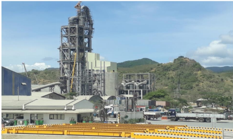
Line 3 Pyro Process Area*
